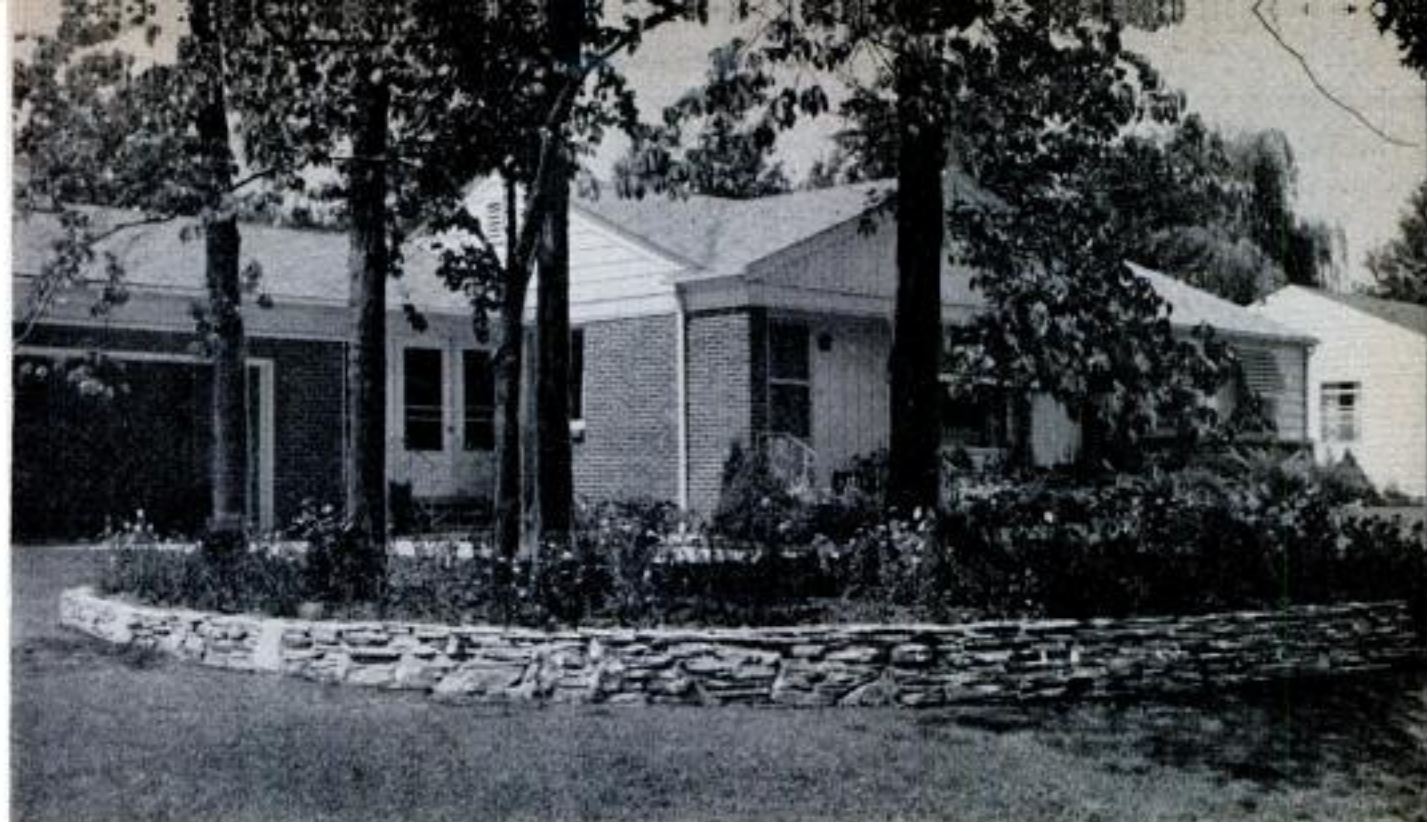
Trees left with roots exposed when lot was graded are saved by island of enriched soil encircled by stone wall
